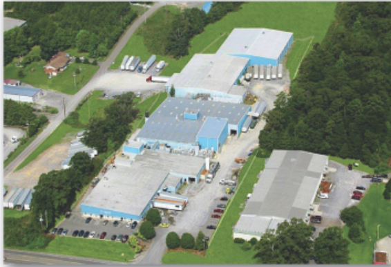
Synalloy Specialty Chemicals – Manufacturers Chemicals Cleveland, Tennessee Facility
